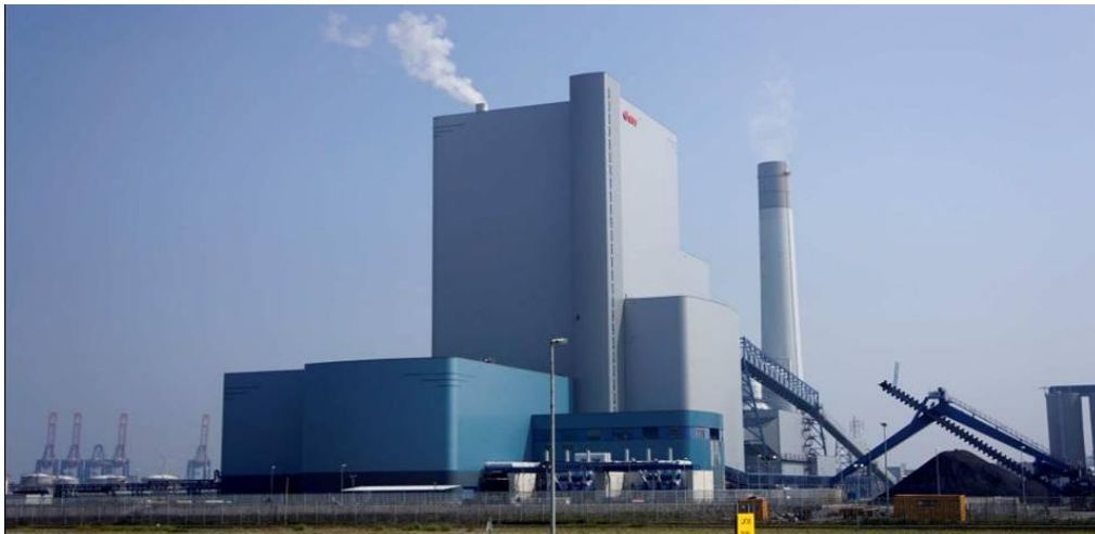
Fig 1: Ultra-Modern Power Plant at Maasvlakte near Rotterdam- MPP3
