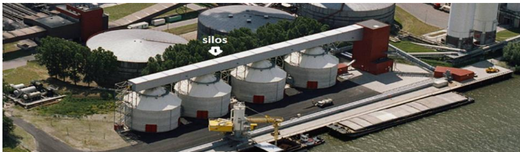
Fig 2: biomass unloading area of Amer power station.
